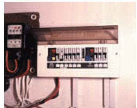
Figure 7.2 Consumer unit in a house.
