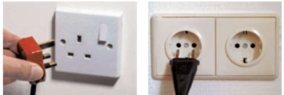
Figure 7.4 Plug sockets in the UK and in Portugal.
