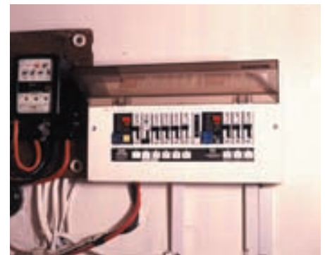
Figure 7.2 Consumer unit in a house.
