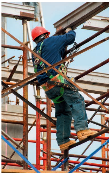
Figure 1.11 Working at height on a building scaffold
