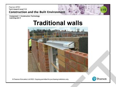
Explain how traditional construction uses walls built out of bricks and blocks. This photograph shows cavity walls with an external leaf in facing bricks and an internal leaf constructed of blockwork. The cavity will be filled with cellulose insulation. You can see the lintels above the window openings to support the brickwork above.
